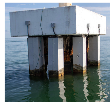
Multi-pier Leg Structure pictured above
