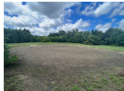
Sweeping view of Lake Jackson Dam #2
